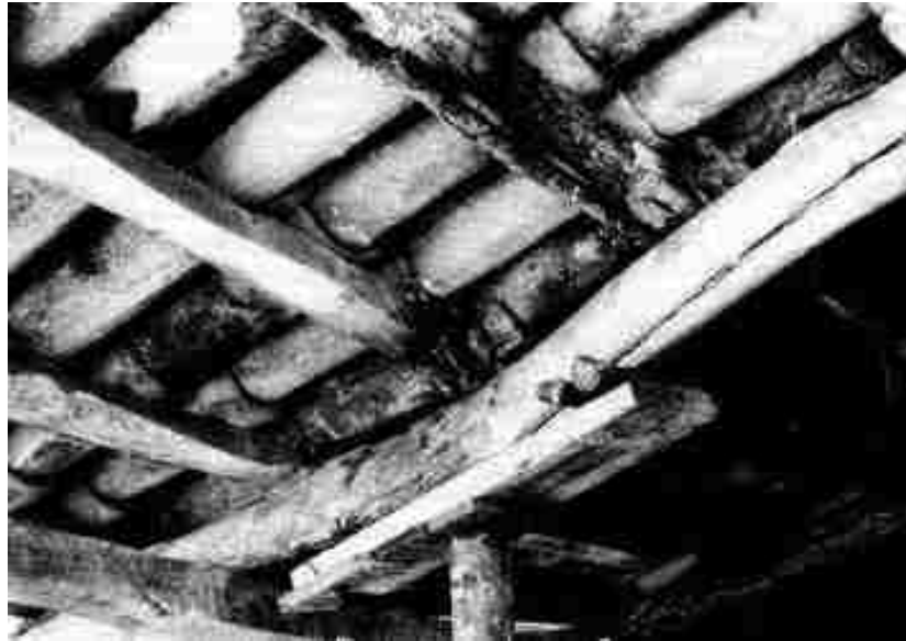
Figure 5.21. Modern tiled roof with tiles resting directly on the rafters (Ö. Wikander 1993:123).
